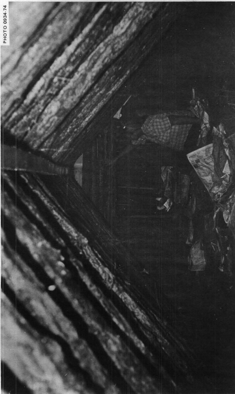
Fig. 5.53. Entrance of the A-Frame Pole Shelter which had a main room 21 ft long and 13 ft wide. It rated a 21-person shelter (as Kearny rated this shelter), this gives each person 13 sq ft of floor space. Both builders and civil defense officials who inspected these shelters agreed that people could get by with 10 sq ft per person of floor space, even though the roof was low and sloping.
